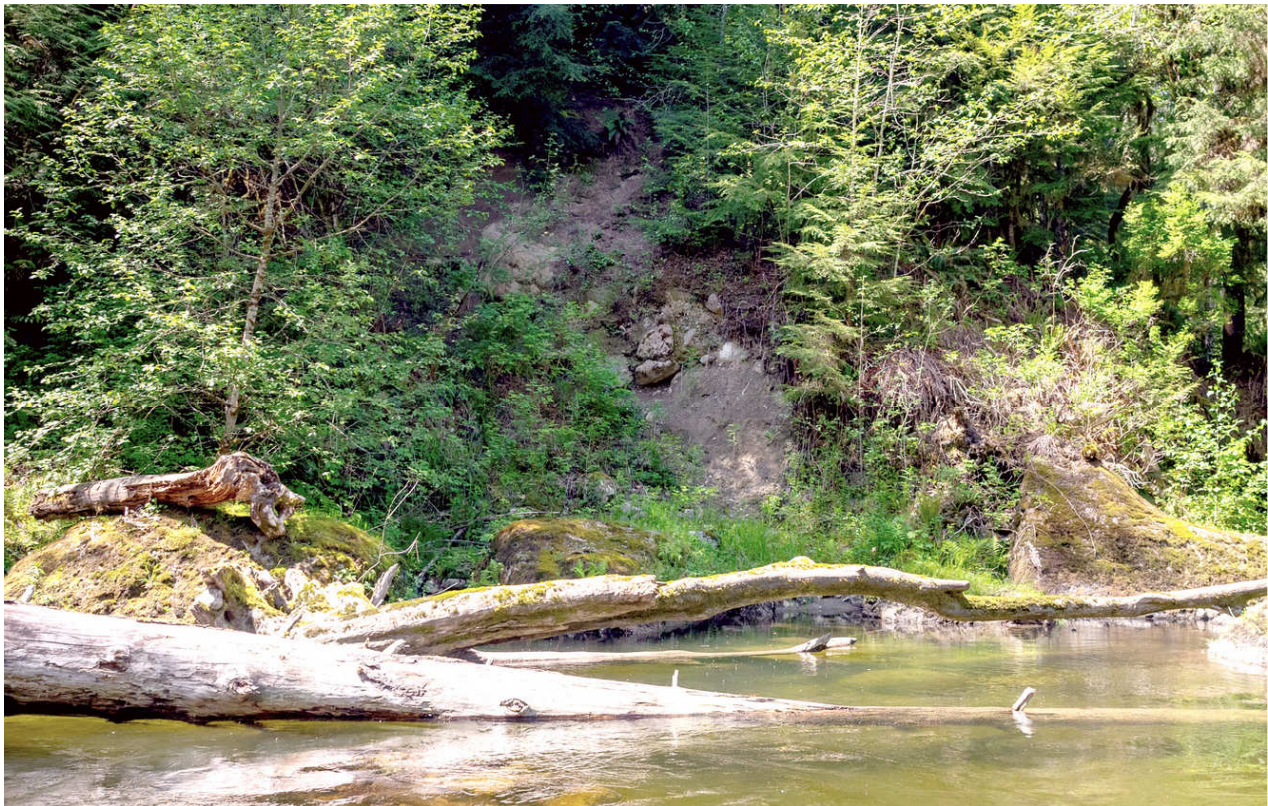
Figure 2. Bank Failure on Outside of Meander Bend (River is cutting a new channel behind the small tree in the foreground.)
